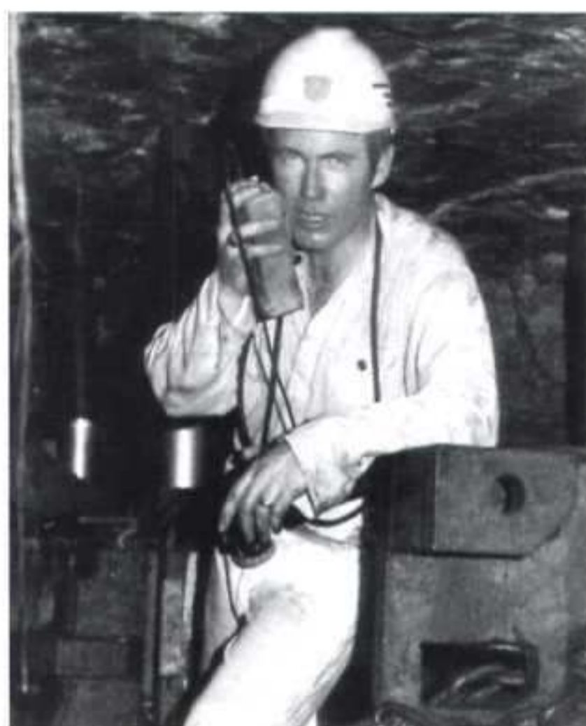
Fig. 7. The 903kHz handheld transceiver being used in a mechanized goldmine stope c.1976
